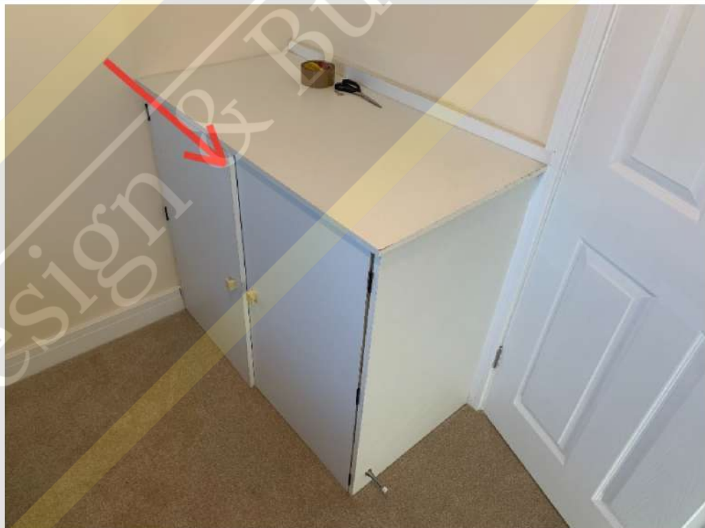
Doors do not close properly and drag on carpet (bedroom 3)
