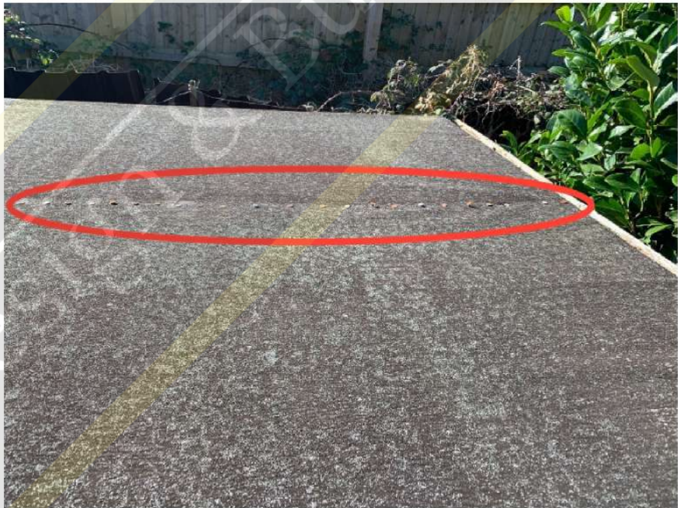
Poorly fixed roof covering
