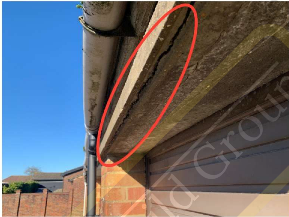
Cracked lintel
