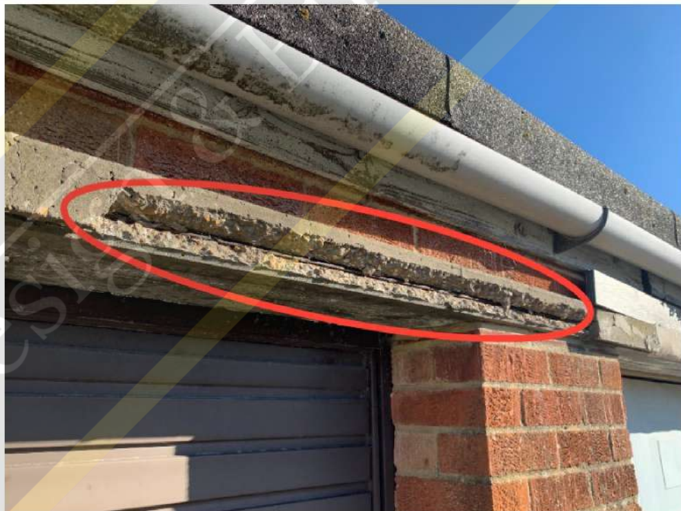
Deteriorated lintel and rusty rebar
