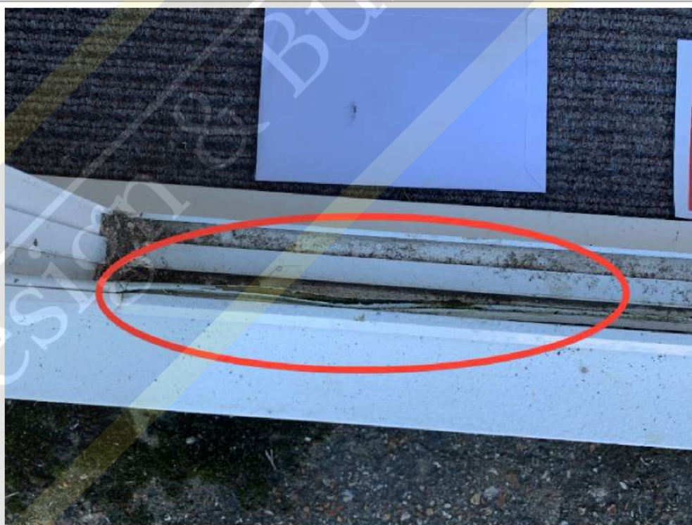
Deteriorated gaskets (front door)
