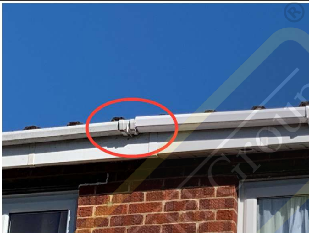
Poorly made joint (rear gutter)
