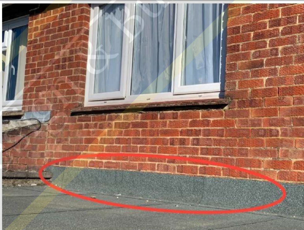
Poorly installed flashing (extension roof)
