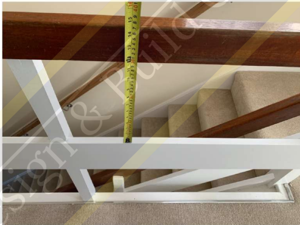
Gap is wider than required
