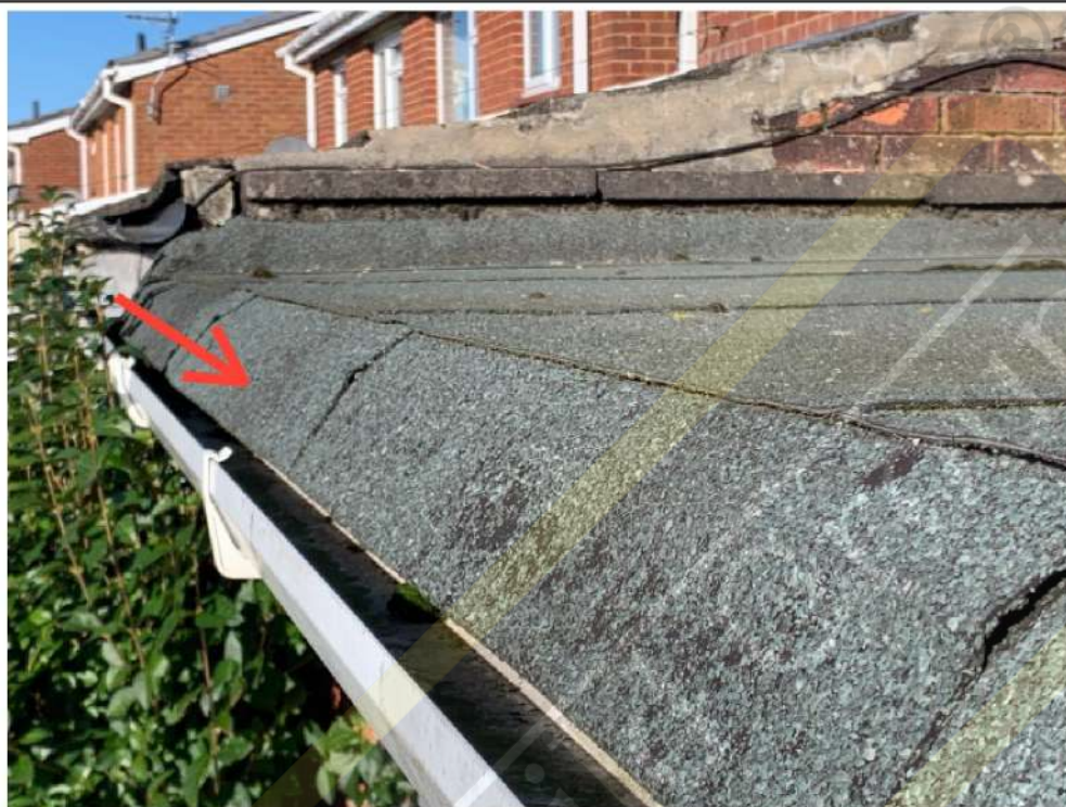
Poorly installed felt
