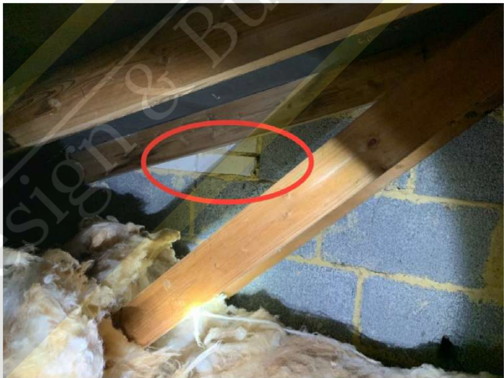
Deteriorated pointing
