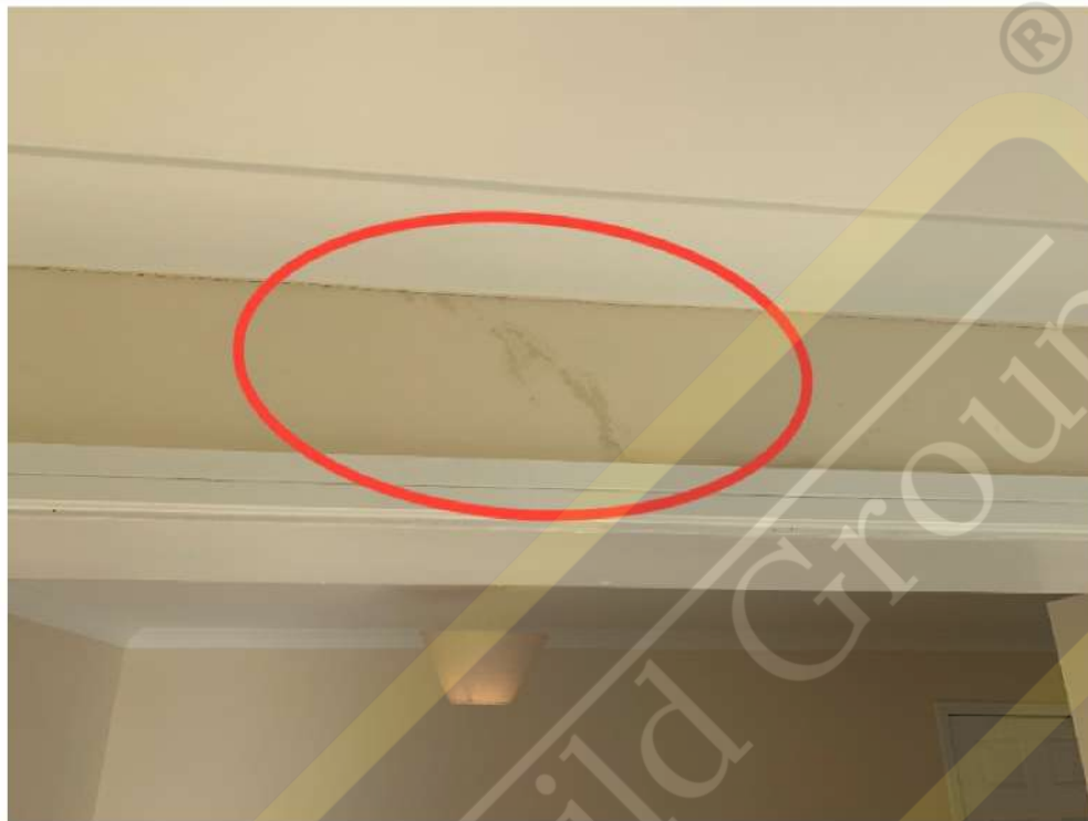
Hairline crack with high moisture content (wall between dining room and kitchen)
