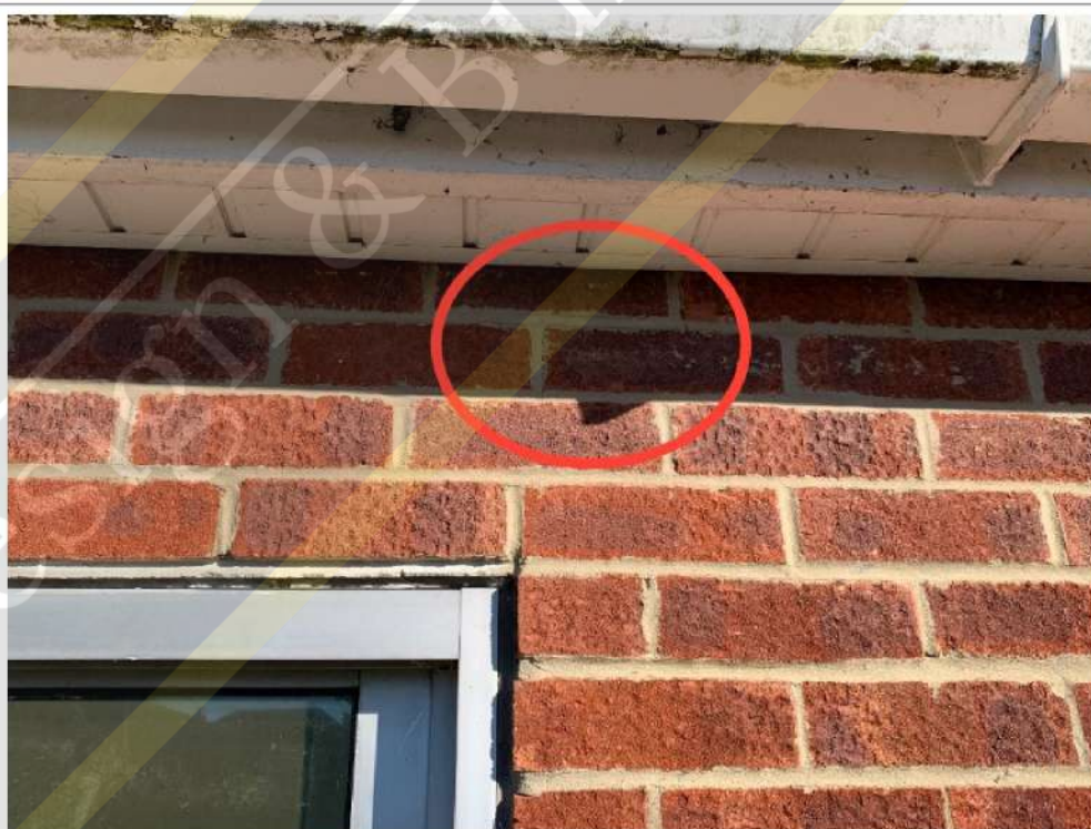
Hairline crack (extension rear wall)
