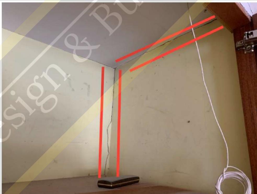
Slight and hairline cracks (bedroom 1 wardrobe)
