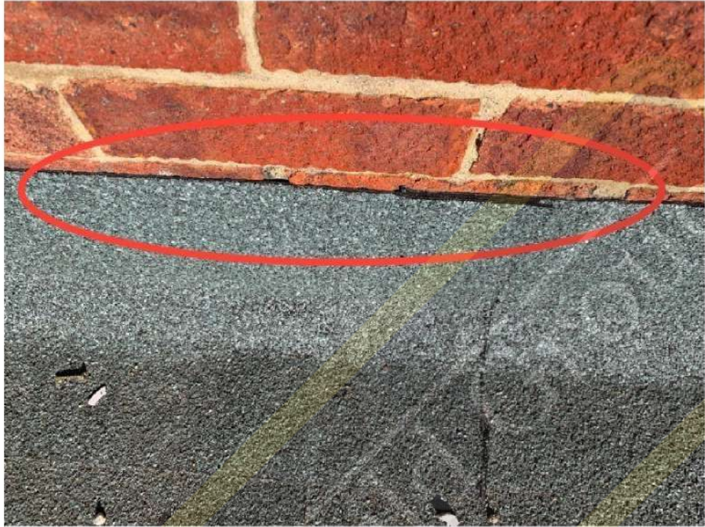
Poorly installed flashing (extension roof)
