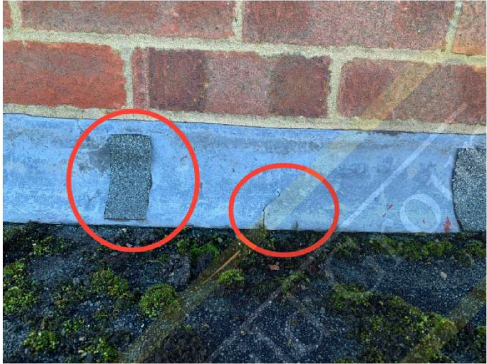
Cracked and poorly repaired flashing (front flat roof)
