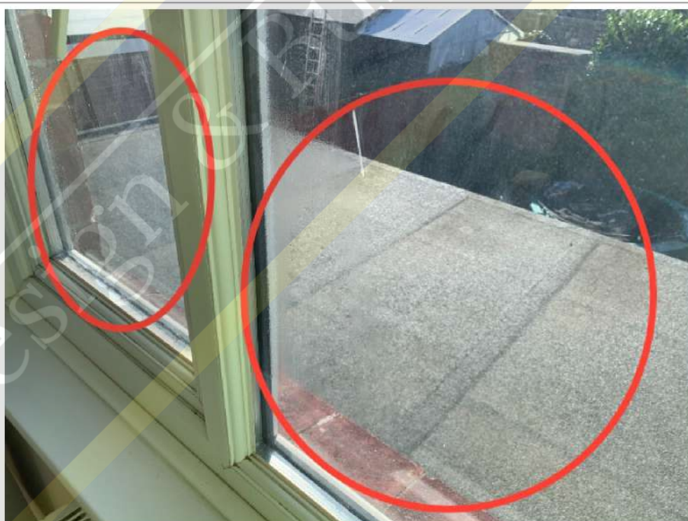
Condensation inside double-glazed units (bedroom 2)
