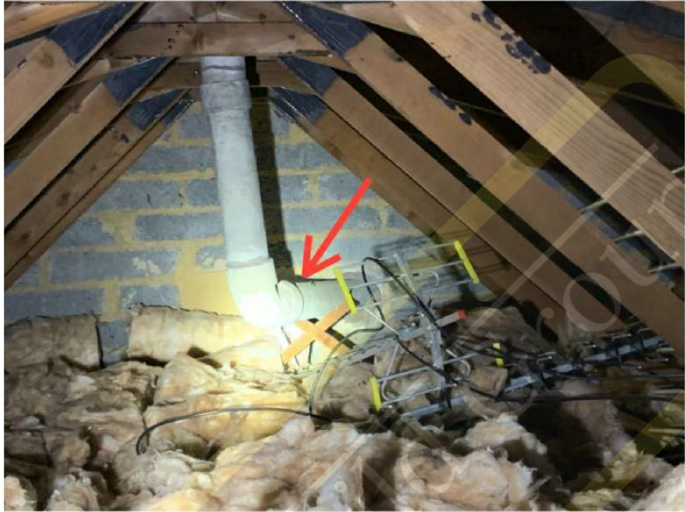
Asbestos cement flue supported by two timber planks
