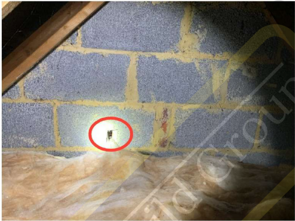
Minor opening in a gable wall
