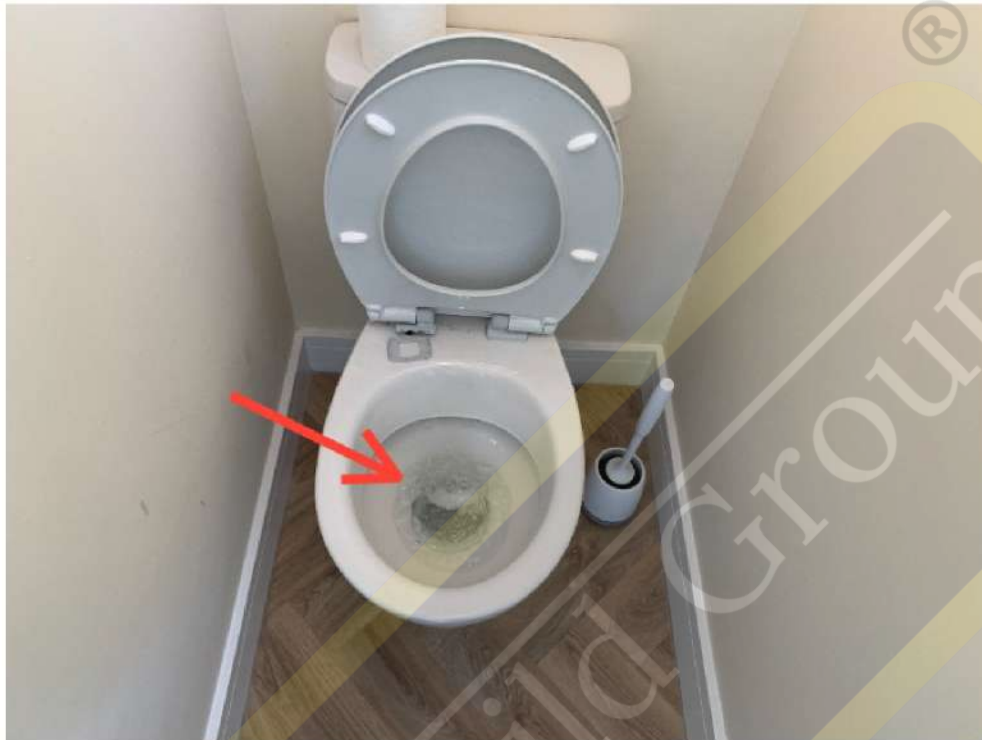
Water does not drain properly
