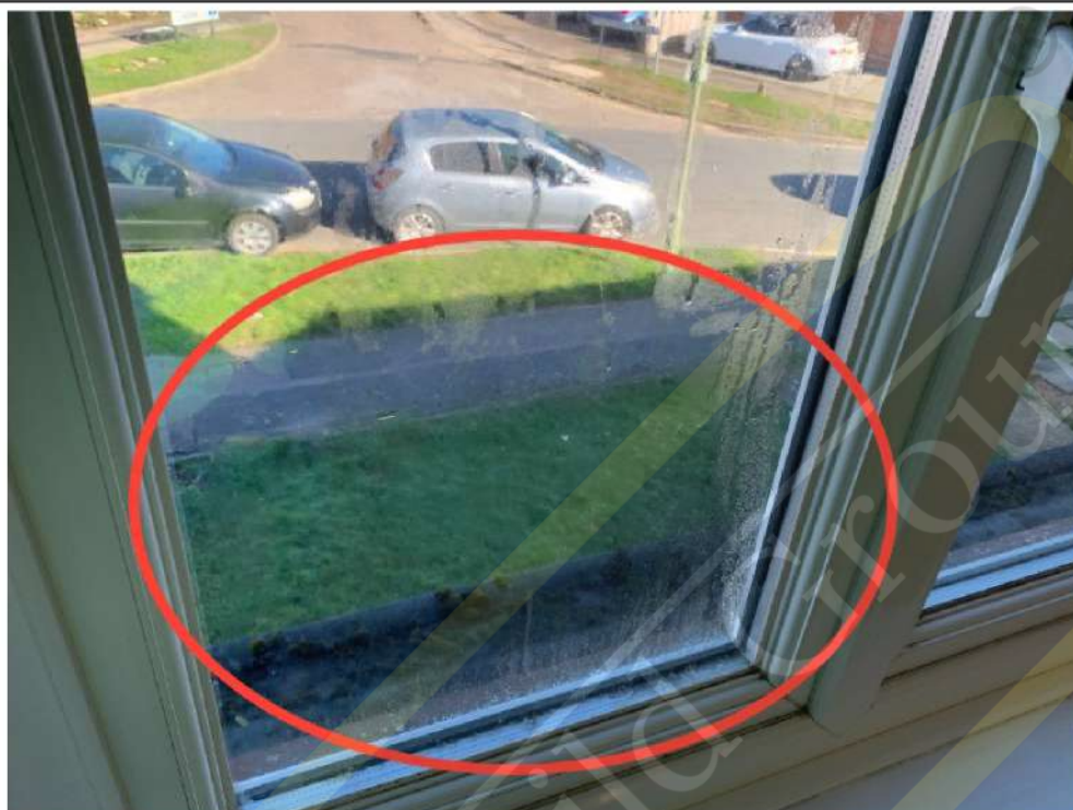
Condensation inside double-glazed unit (bedroom 1)
