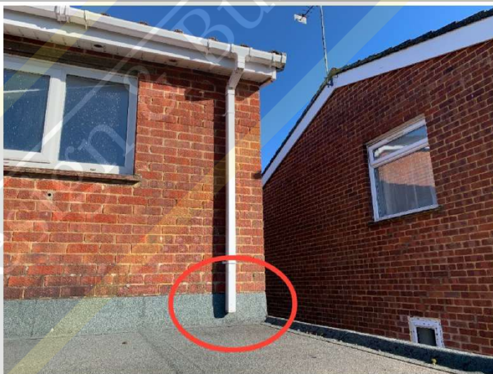
Downpipe from main roof discharges onto extension roof
