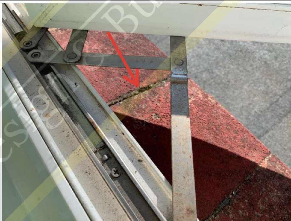
Window sill deteriorated pointing (rear bedroom window)
