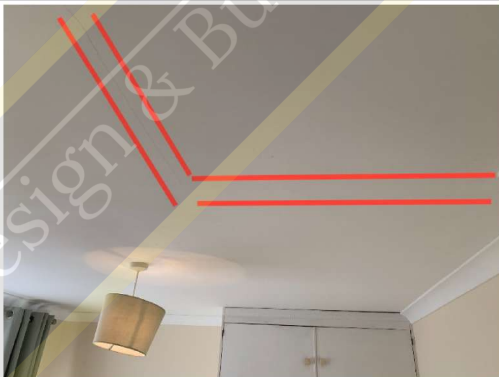
Hairline cracks in plasterboard ceiling (bedroom 2)
