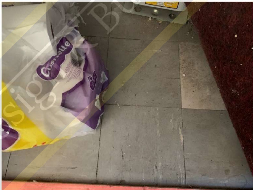
VAT tiles (cupboard under the stairs)
