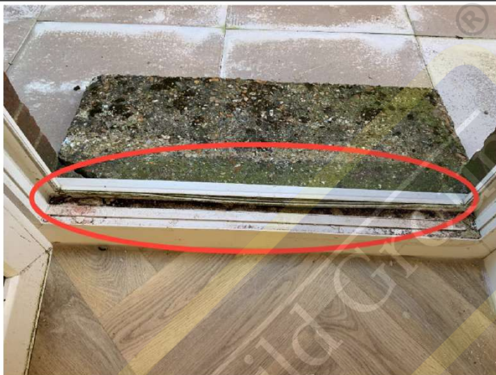
Deteriorated gaskets (side door)
