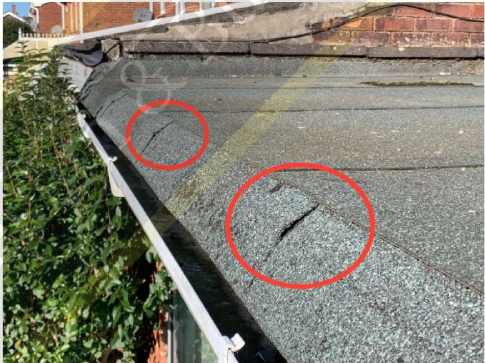
Deteriorated felt (extension roof)
