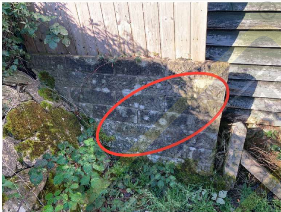
Cracks in the boundary wall
