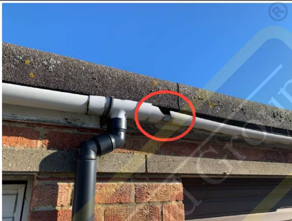
Broken gutter
