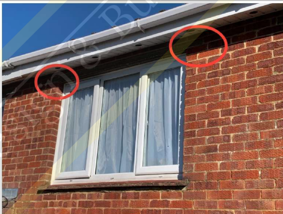
Cracks above window (rear wall)
