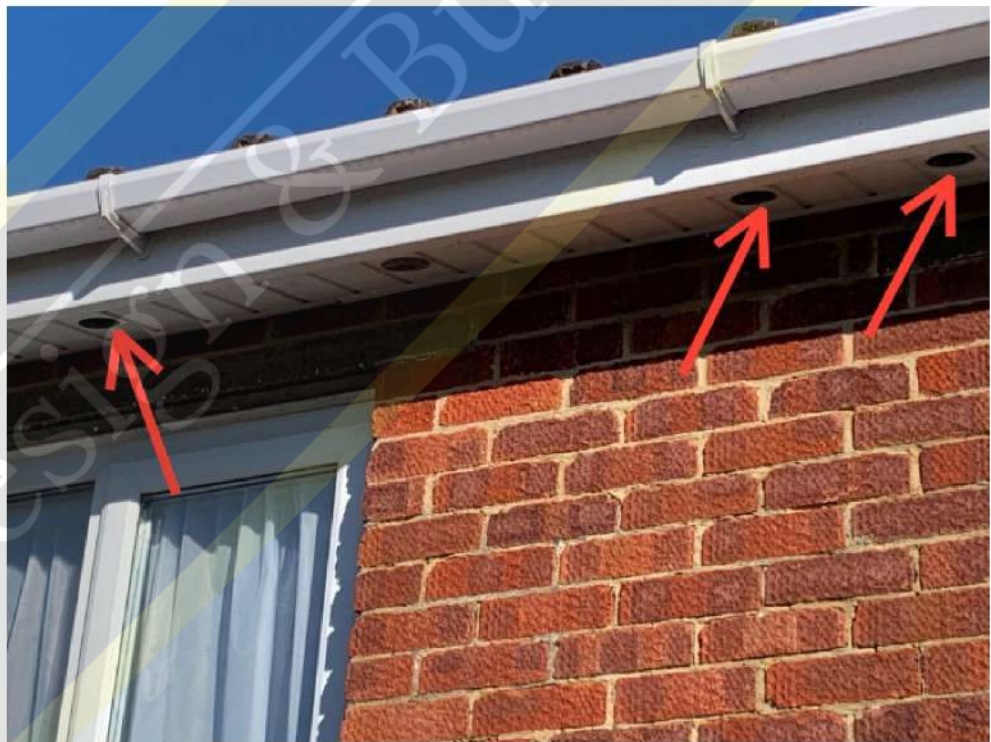
Missing soffit vent grills
