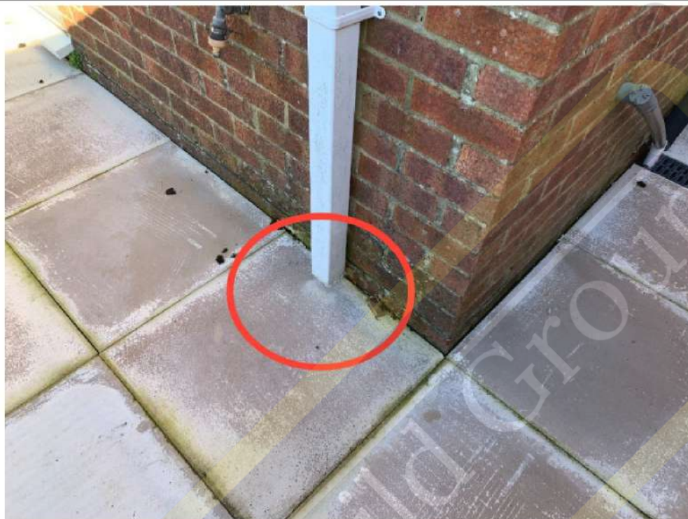
Rear downpipe discharges onto the ground
