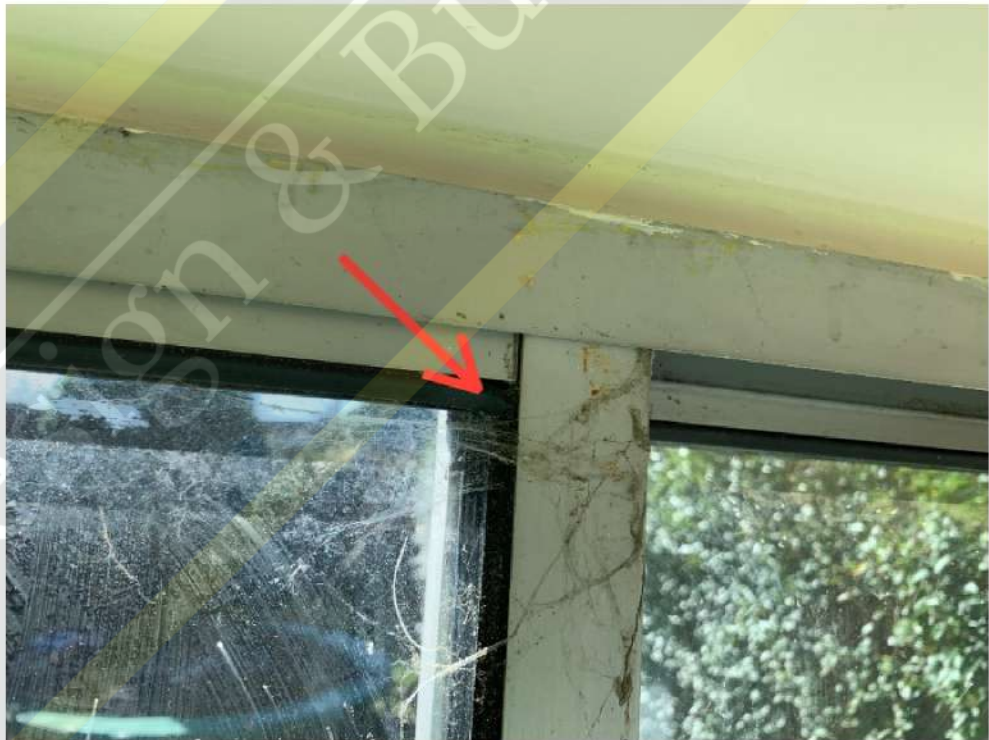
Deteriorated gaskets (rear door)
