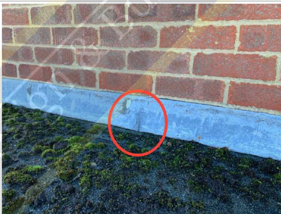
Cracked flashing (front flat roof)
