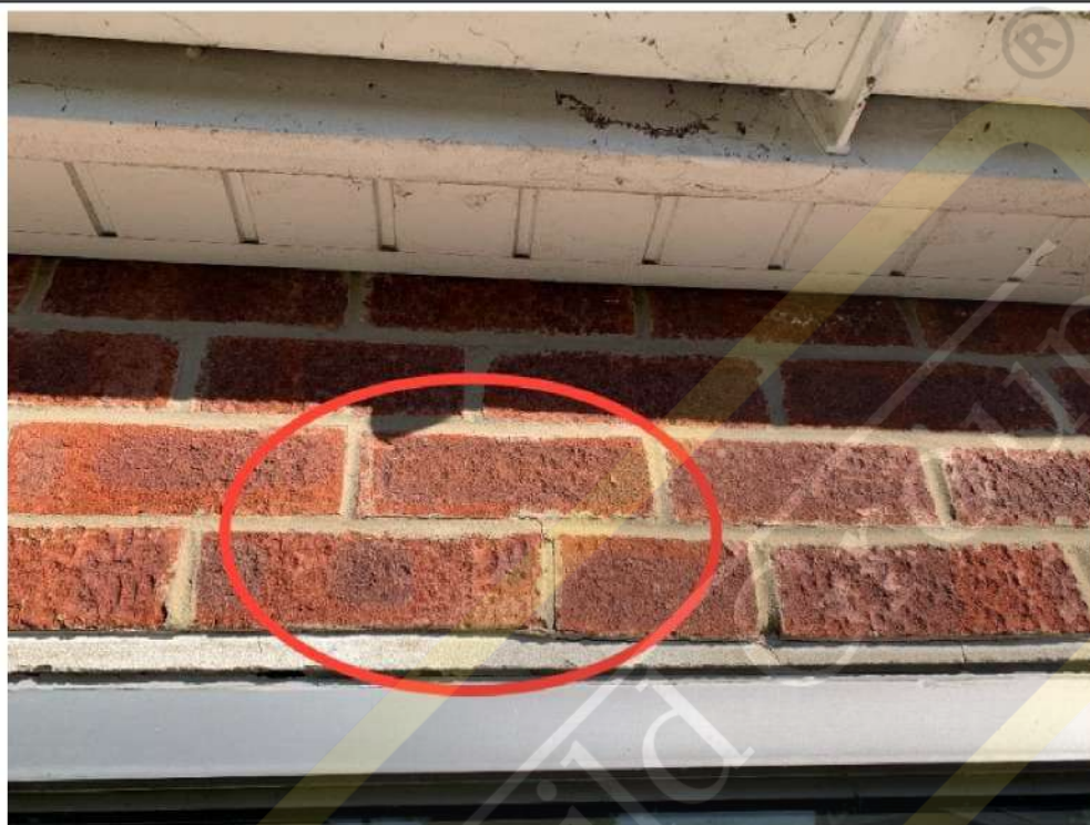
Hairline crack above the rear door (extension rear wall)
