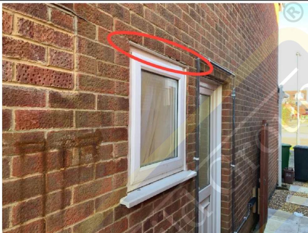
Deteriorated pointing (side wall)
