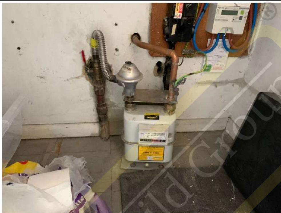
Gas meter (cupboard under the stairs)
