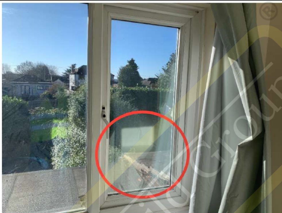
Condensation inside double-glazed unit (bedroom 2)
