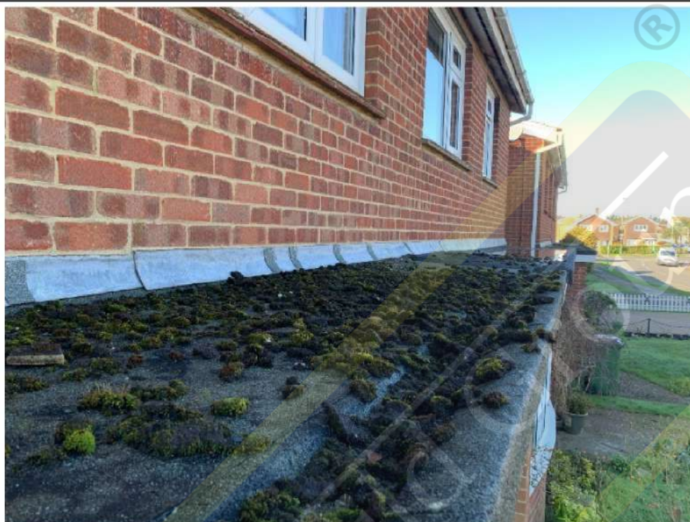
Moss growing on flat roof (front flat roof)
