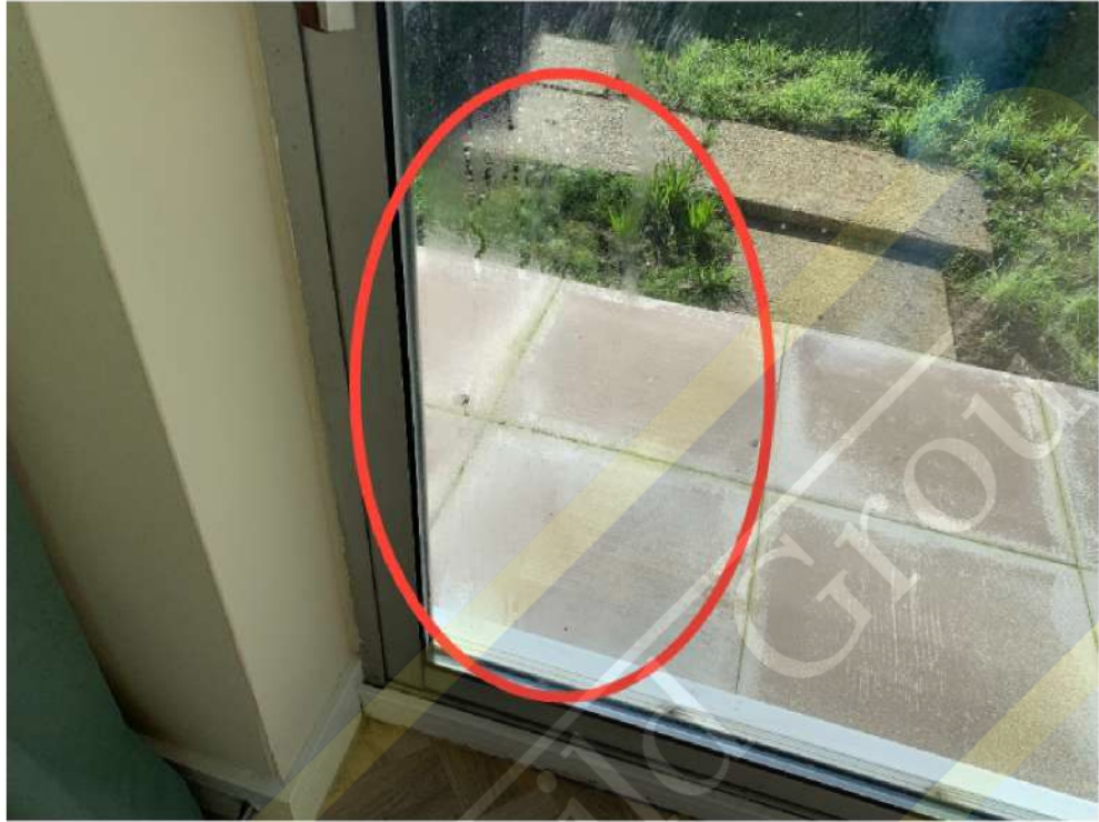
Condensation inside large double glazed unit (rear door)
