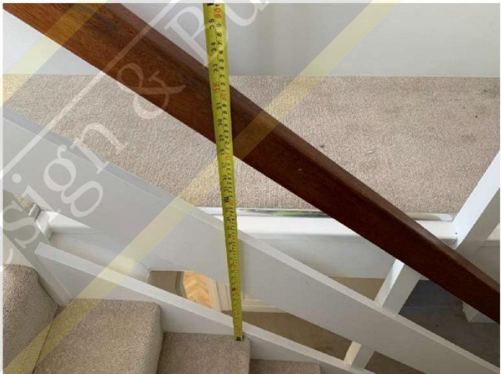
Handrail is lower than required
