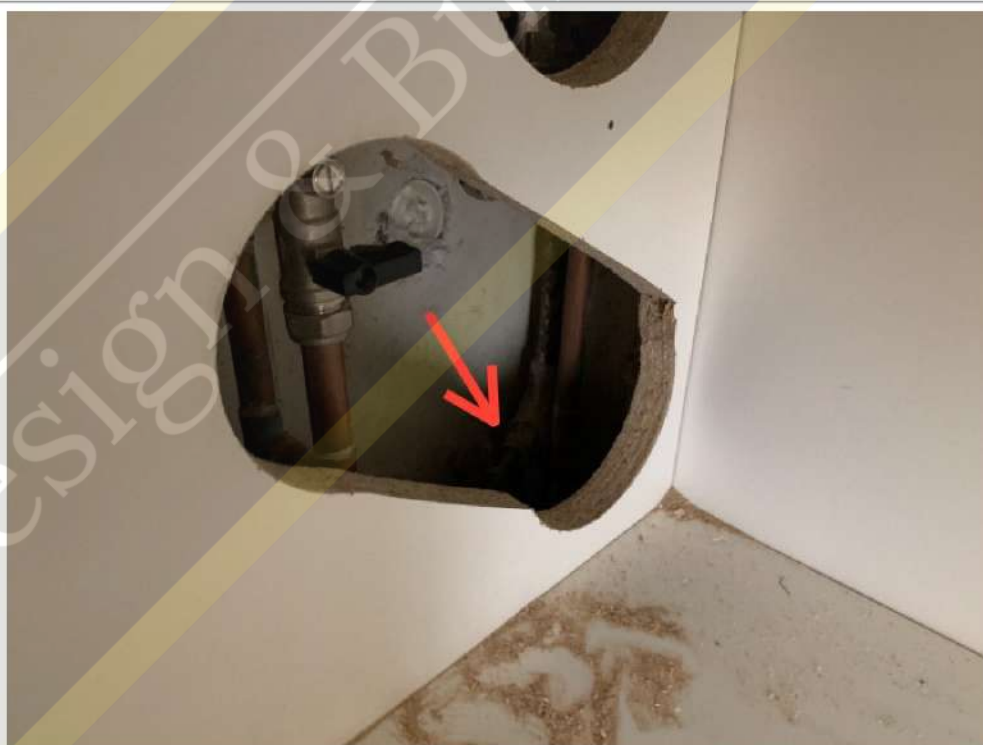
Internal stop tap (kitchen corner unit)
