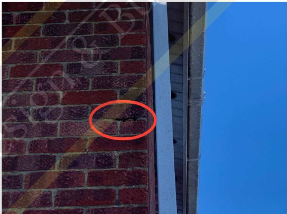
Deteriorated pointing (side wall)
