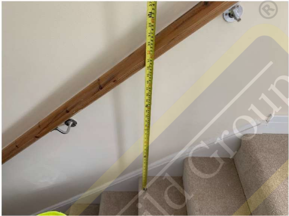
Handrail is lower than required
