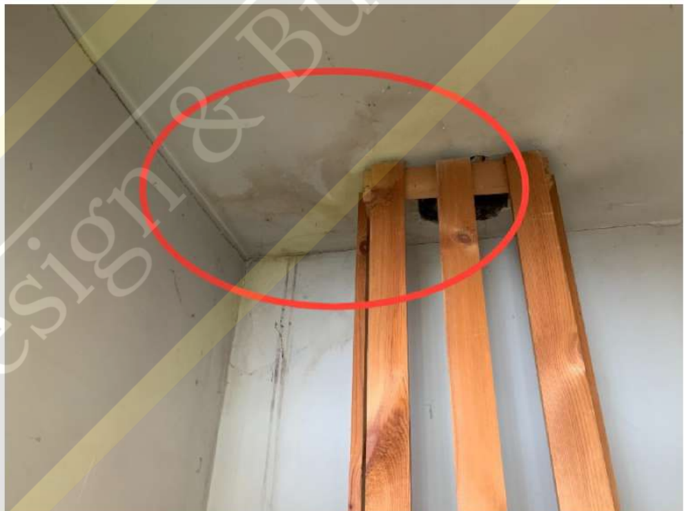
Leak stains (landing cupboard)
