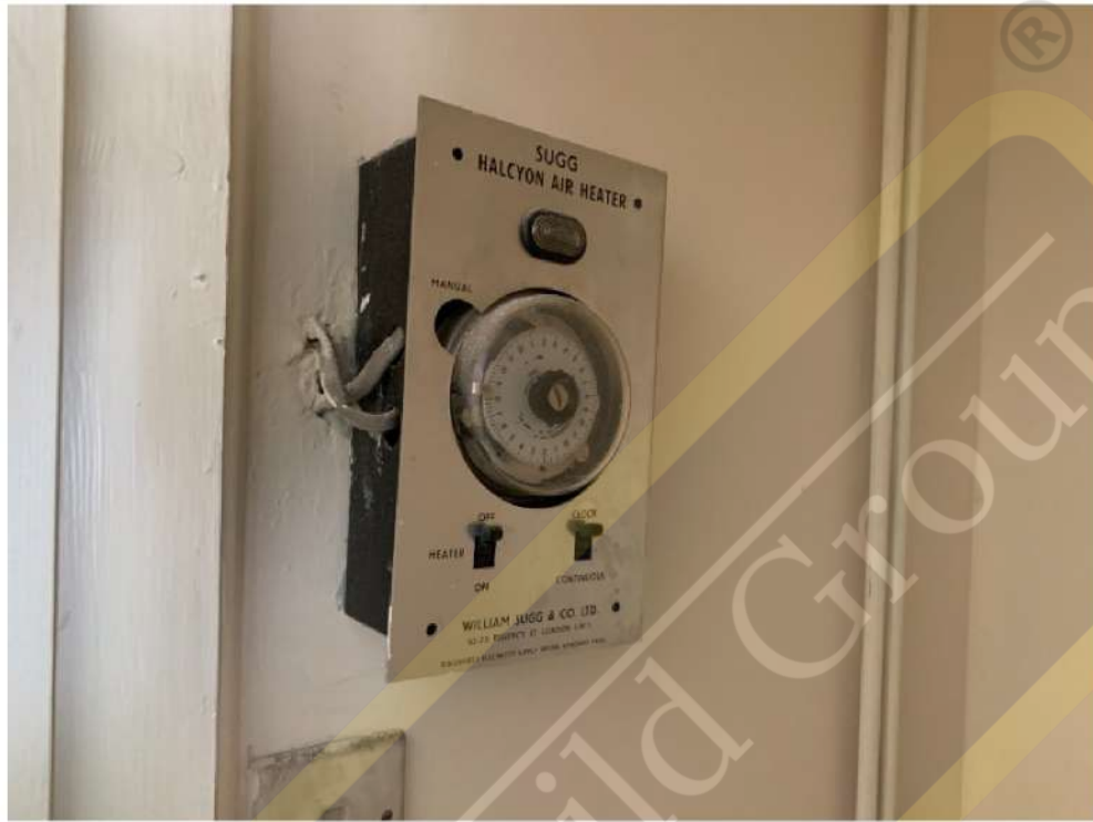
Old air heater control panel
