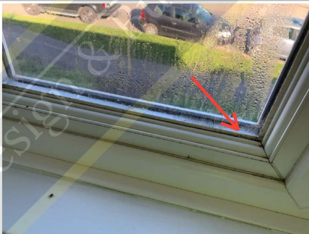
Mouldy and deteriorated gaskets (bedroom 1)
