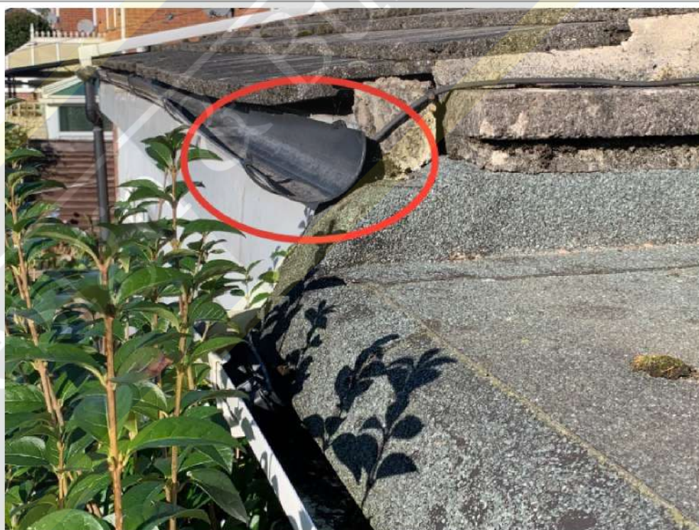
Neighbour's gutter stop end is missing
