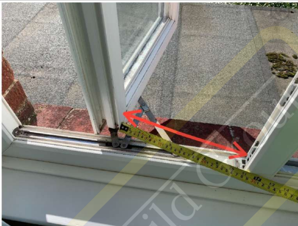
Unobstructed opening is less than required (rear bedroom)
