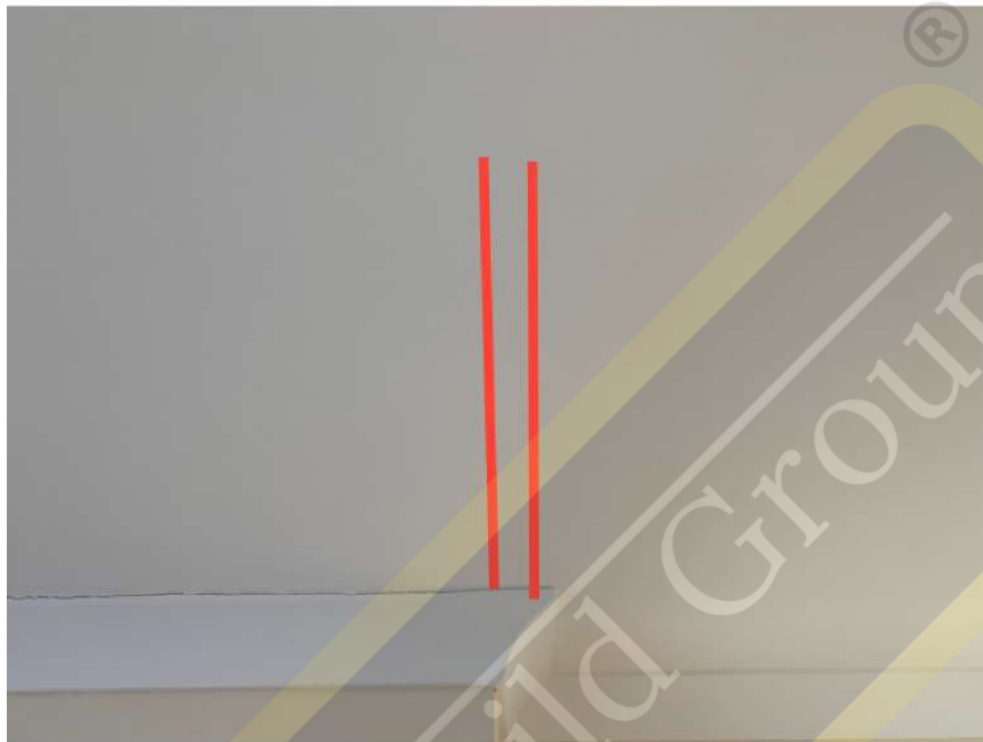
Hairline crack in plasterboard ceiling (bedroom 1)
