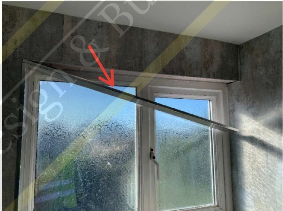
Detached plastic wall panel (bathroom)
