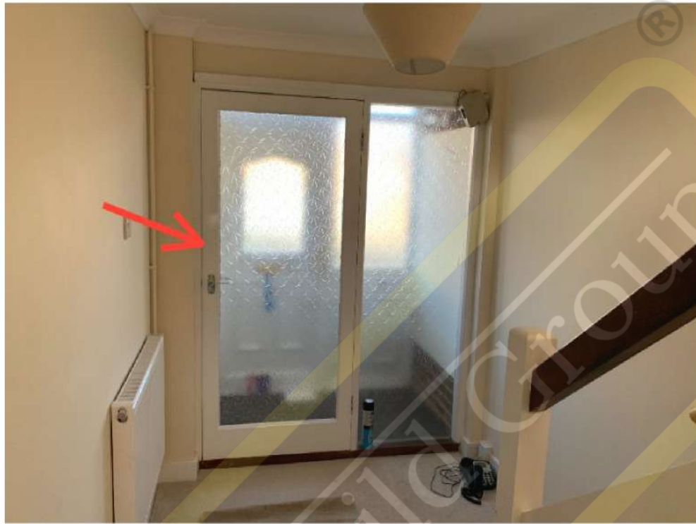
Door does not close properly (hallway)
