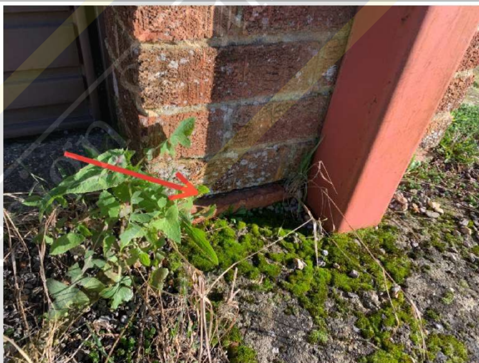
DPC is lower than 150 mm from the ground
