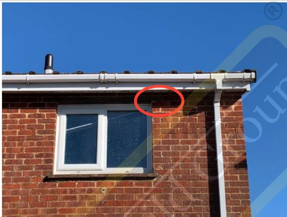
Crack above window (rear wall)
