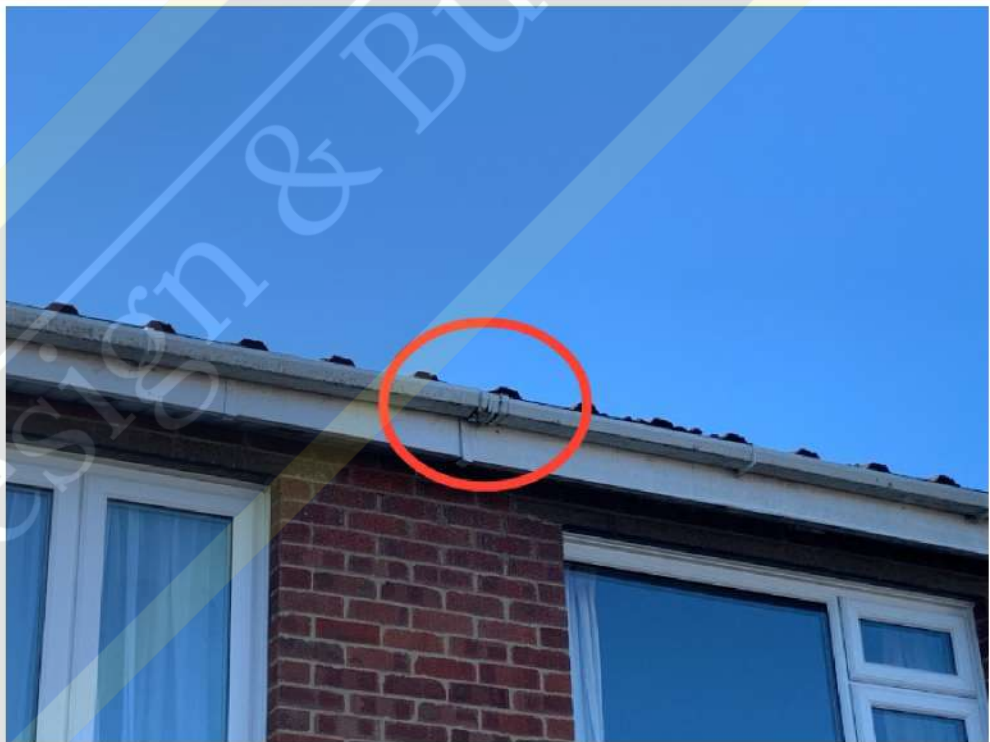
Poorly joint (front gutter)
