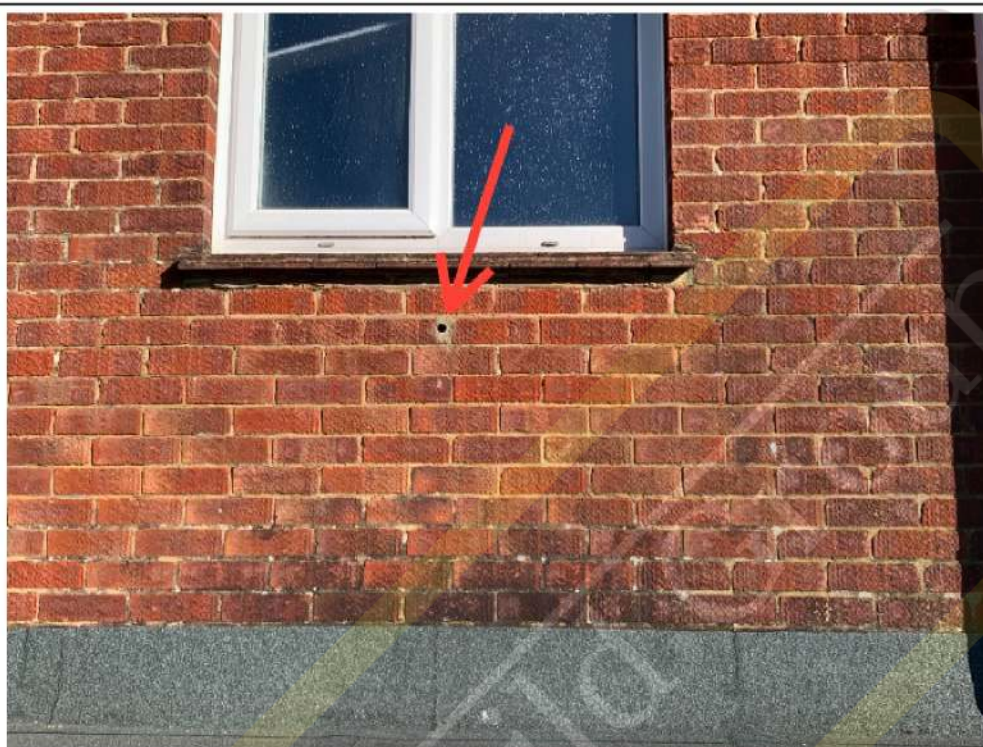
Unused service hole (rear wall)
